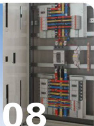
TỦ DB Distribution Board ( DB )
